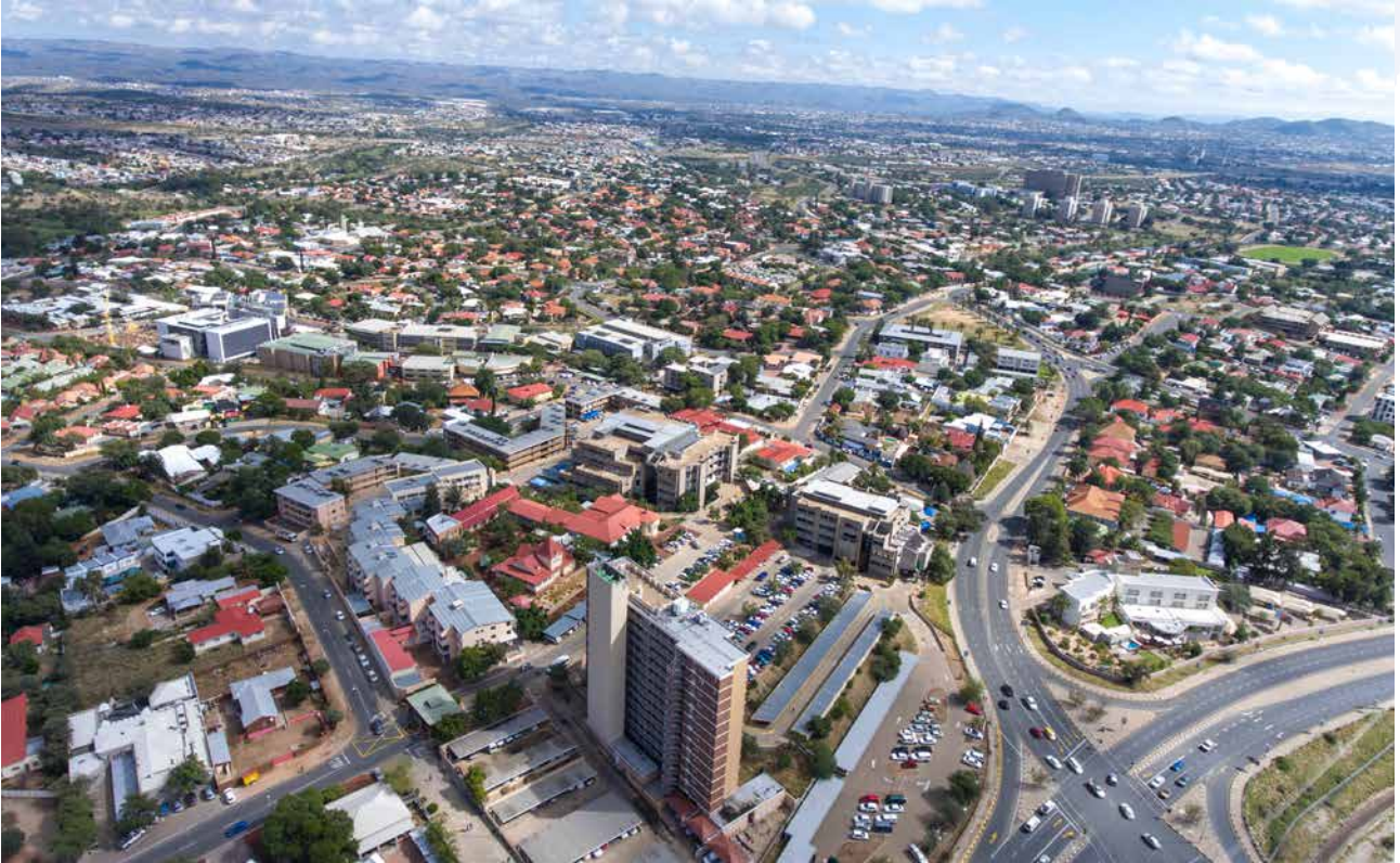
A view of Windhoek, the capital of Namibia. Urbanisation in Namibia is affected by population dynamics in urban population growth and internal migration, rural poverty that causes people to migrate to the city to improve their livelihood and re-gazetting of some urban areas. Photo © NUST.
