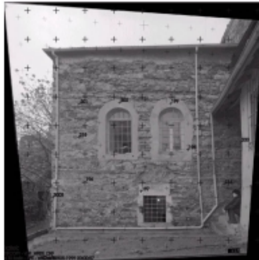
Figure 3. Rectified image of the facade of Dimitri House by photogrammetric software.
