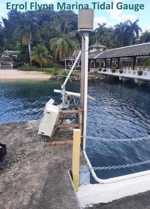
The Errol Flynn Marina has an acoustic and Radar sensor. The tall pole is the acoustic and radar sensor overhang the water.
