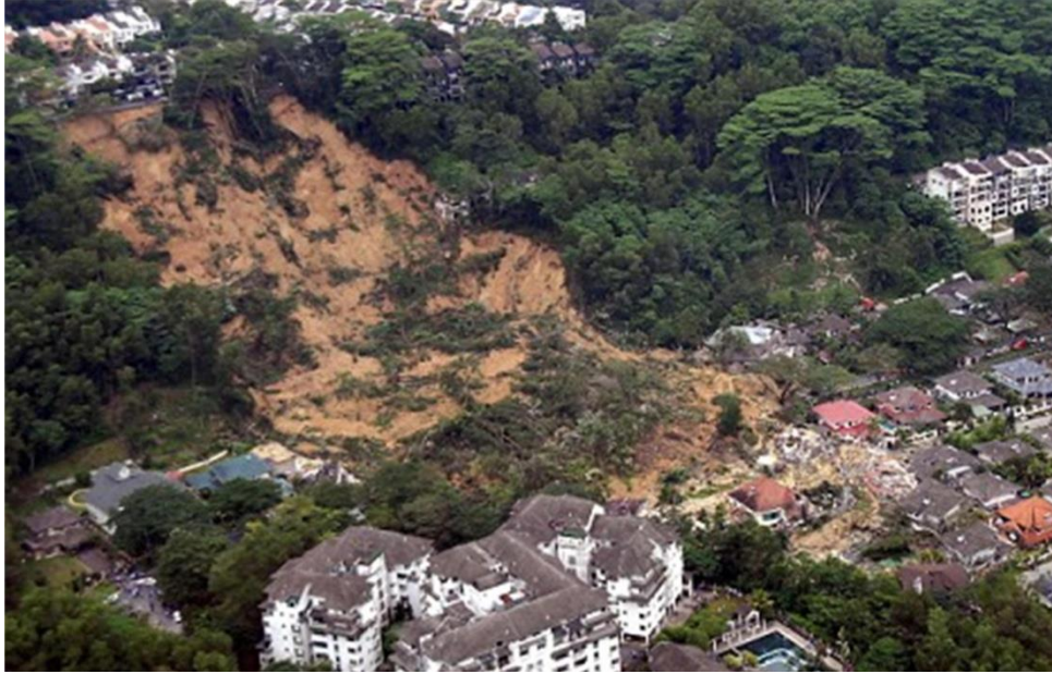
Figure 1: The leakage pipe had caused the landslide tragedy at Ulu Klang, Kuala Lumpur, Malaysia.
