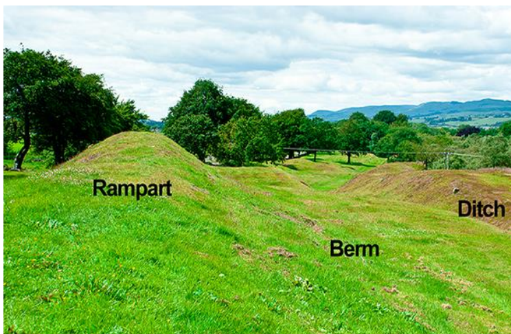
Fig. 3 Typical view of the design of the Antonine Wall showing the rampart, berm and ditch as it crosses the countryside.
