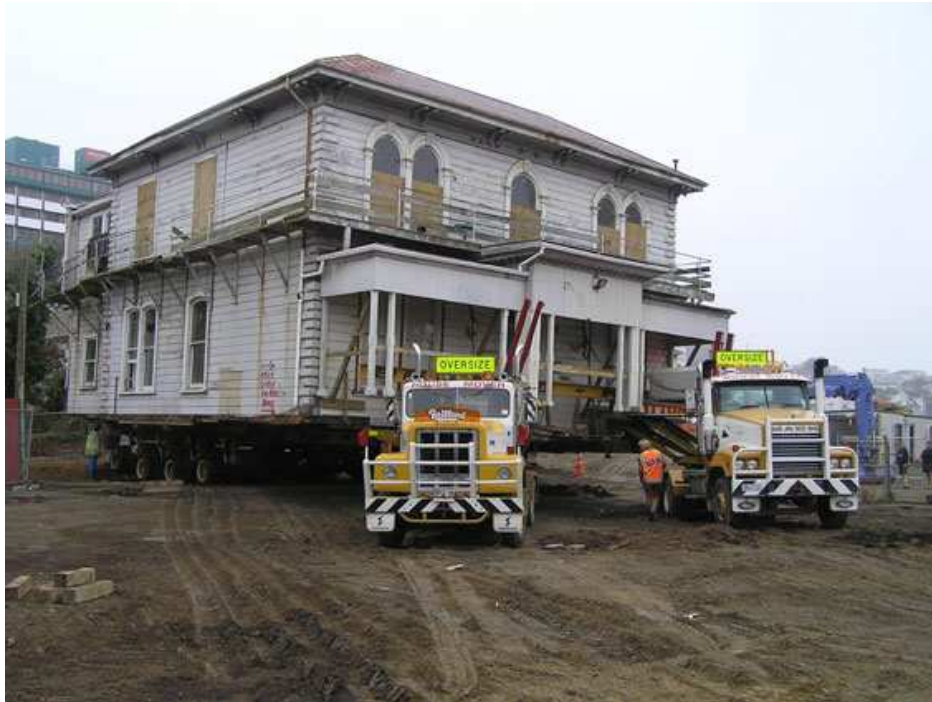
Figure 6: Floodplain building relocation in Illinois, USA (Source: http://www.lakecountyil.gov/Stormwater/LakeCountyWatersheds/BMPs/PublishingImages/building_relocation.jpg ).
