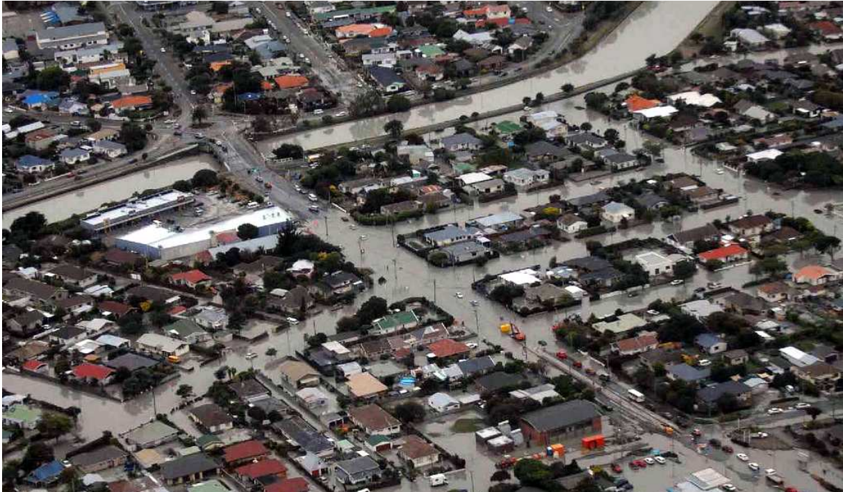
Figure 2: Christchurch (New Zealand), flooded areas after earthquake (Author: New Zealand Defence Force, http://en.wikipedia.org/wiki/2011_Christchurch_earthquake (last access: 2011-04-09)).
