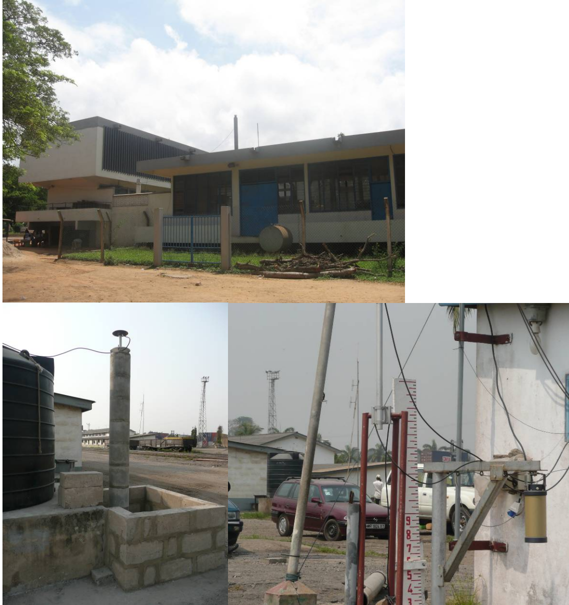
Figure 2 – Details of the installed GNSS stations in Takoradi: TADI station installed by SDG (above); TKTG station installed by CGUL/IDL-SDG-BRRI (below left) and position of TKTG with respect to the tide-gauge (below right).
