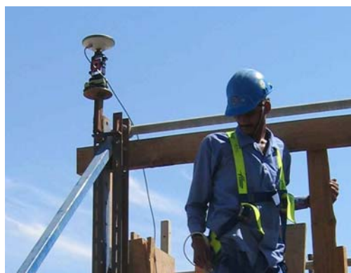
Figure 1: GPS and circular prism collocated
