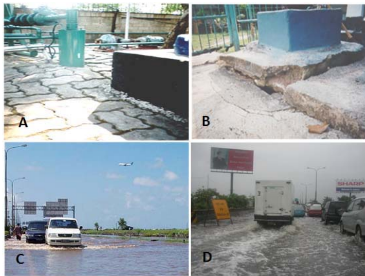
Figure 11. Several indication and impact of land subsidence in Jakarta [Wirakusumah, 2008]. A and B are locations in Kamal Muara; C and D are locations along the highway to the airport (Cengkareng).
