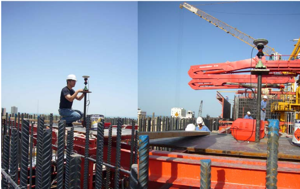
Fig 8: Soang Hoon setting up “Active Control Points” in Kuwait
