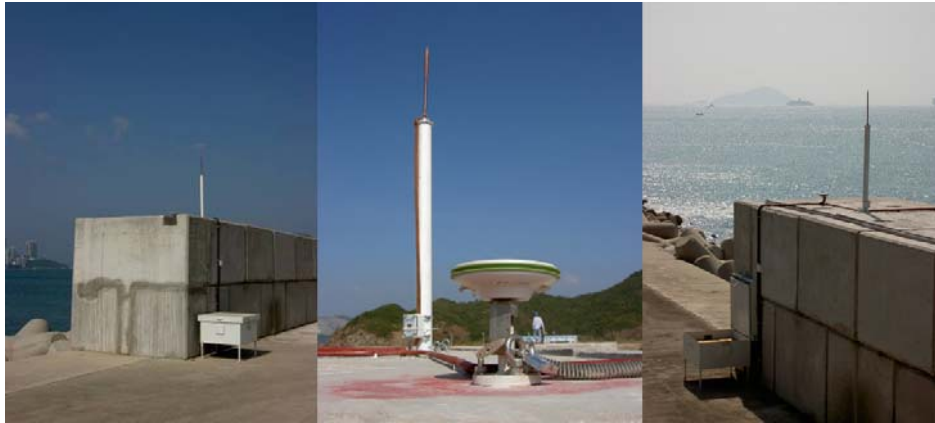
Fig 1: GPS monitoring antenna installed on a sea wall in Hong Kong.
