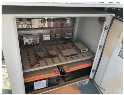
Figure 2: : KSA-CORS IP66 Internal Cabinet filled with Dust
