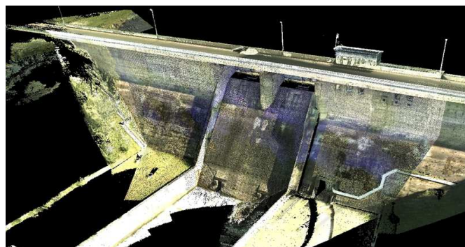
Fig. 3. Results of dam scanning from the windy side.
