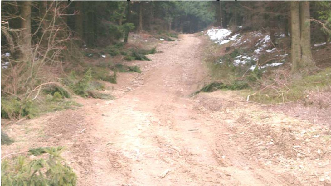
**Figure 3:** This road in the Sauerland-area can only be used for skidding, for trafficability with lumber trucks it needs an adequate induration and width.
