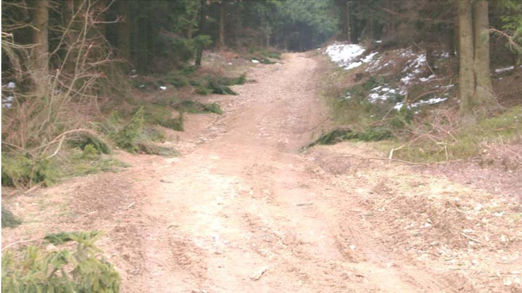
**Figure 3:** This road in the Sauerland-area can only be used for skidding, for trafficability with lumber trucks it needs an adequate induration and width.
