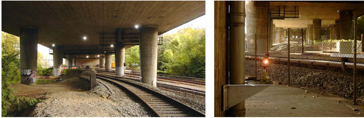
Fig. 6: Impressions from under the bridge
