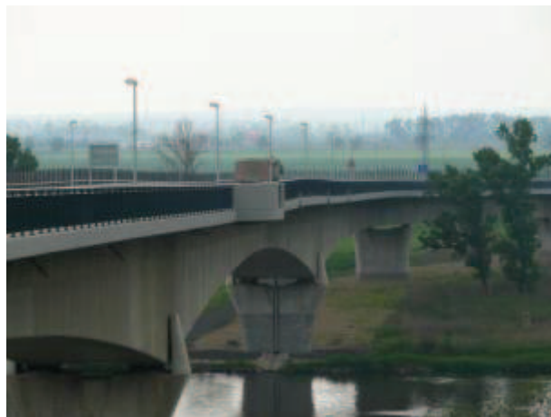
Figure 1c The bridge near Litoměřice
