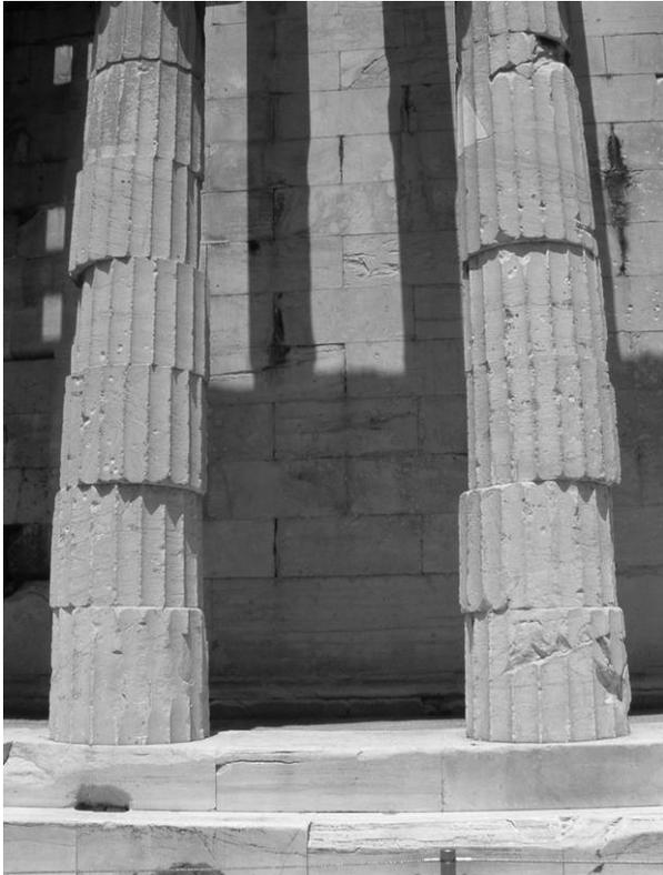
Fig.1 - Sinusoidal offset of the column drums indicative of seismic deformation in the Hephaisteion (Theseion), Athens according to Galanopoulos (1956).
