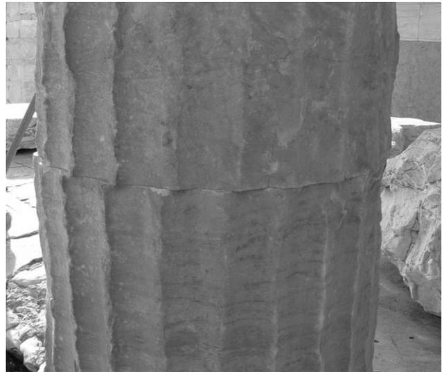
Fig. 2 - Characteristic rotation in the column drums of the Propylaea after the 1999 Athens earthquake.
