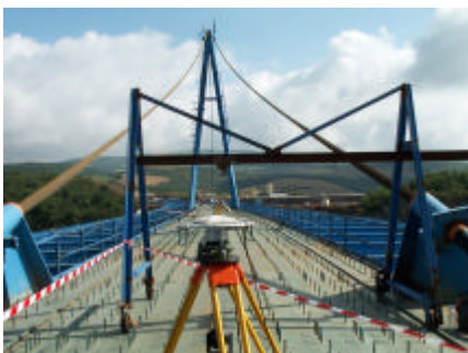
View of point n° PT32
