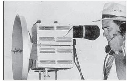
Dr Wadley with the prototype Tellurometer
