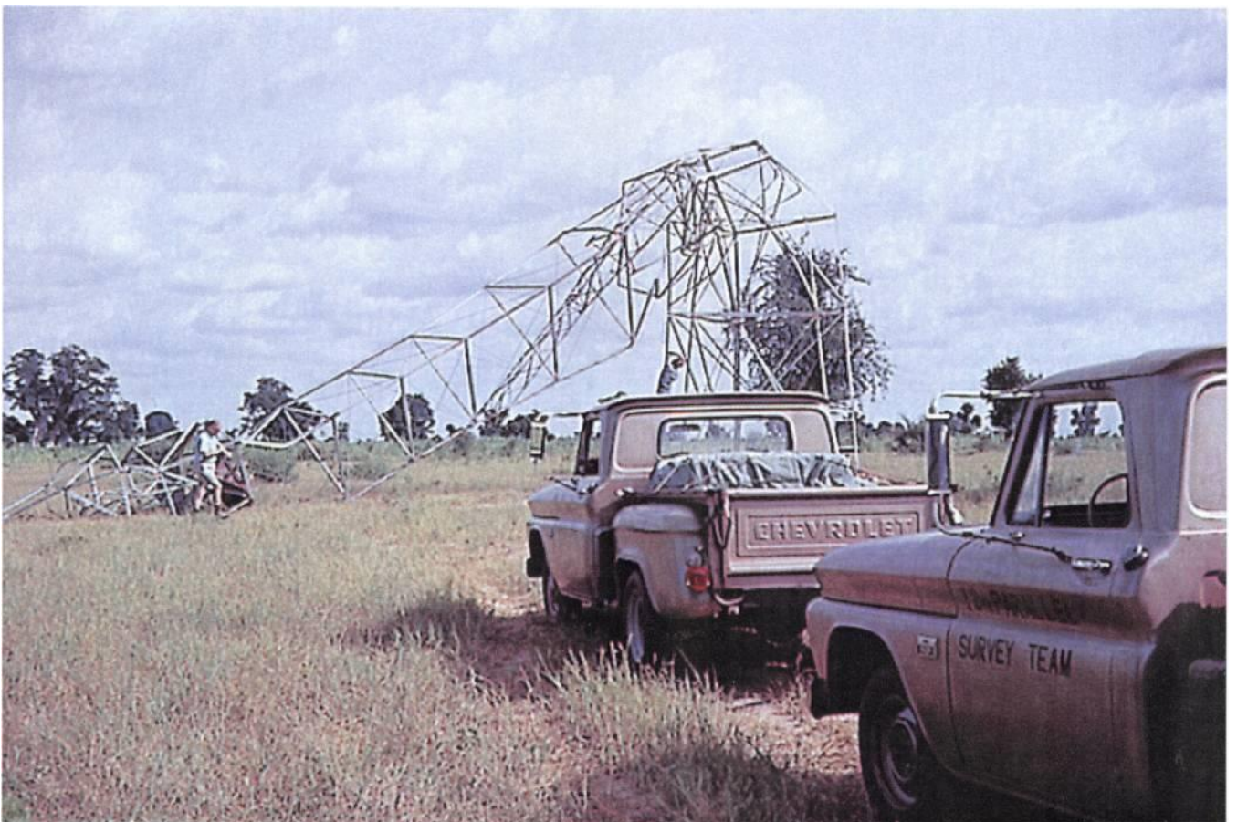
A crumpled Bilby tower near Damaturu. Northern Nigeria, 1969. (Malcolm Anderson)
