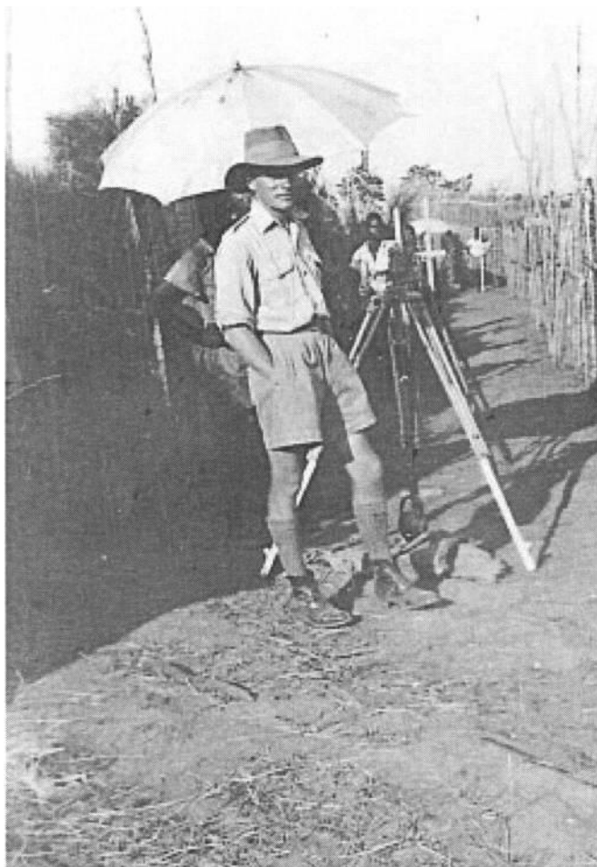
Walter Smith on base-line standardisation. The subsequent measurement was done at night. Nyasaland, 1948.
