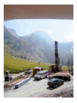
The activities started at the beginning of the year 2000 and will be finished within the end of 2001. Their aim is to determine the most favourable course of the tunnel from a geological/geo-mechanical point of view, allowing an accurate estimate of times, prices and risks related to the construction of the work.
