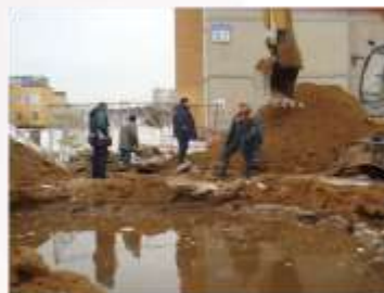
Old engineering infrastructure
