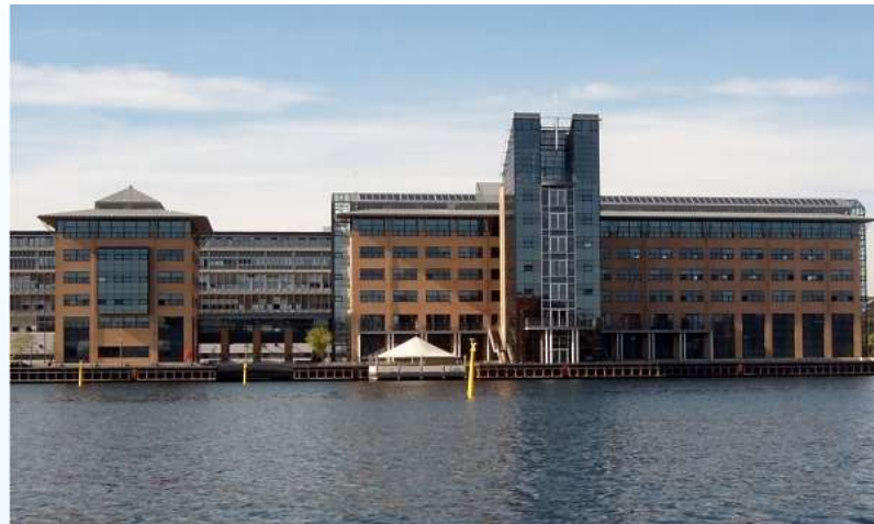
Complex housing the FIG Office, Copenhagen
