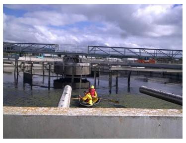
The violent uplift caused by the earthquake fractured these tanks and our task was to determine the extent of damage.
