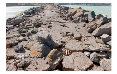
Fingers and breakwaters suffered greatly as they were surrounded by water and although heavily armoured with rock, collapsed into the harbour muds. These were temporarily abandoned until other more important issues had been attended to.
