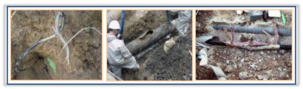
Figure 1: Damage utilities due to excavation works
