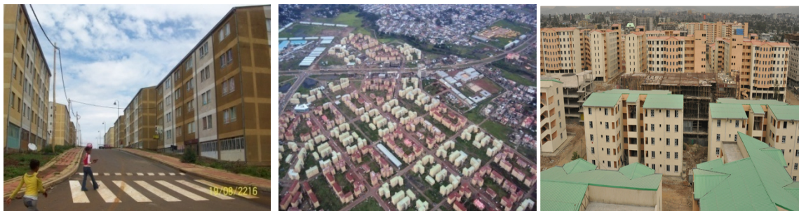
Pic 1: Pictures of some of the apartments completed and transferred to residents
