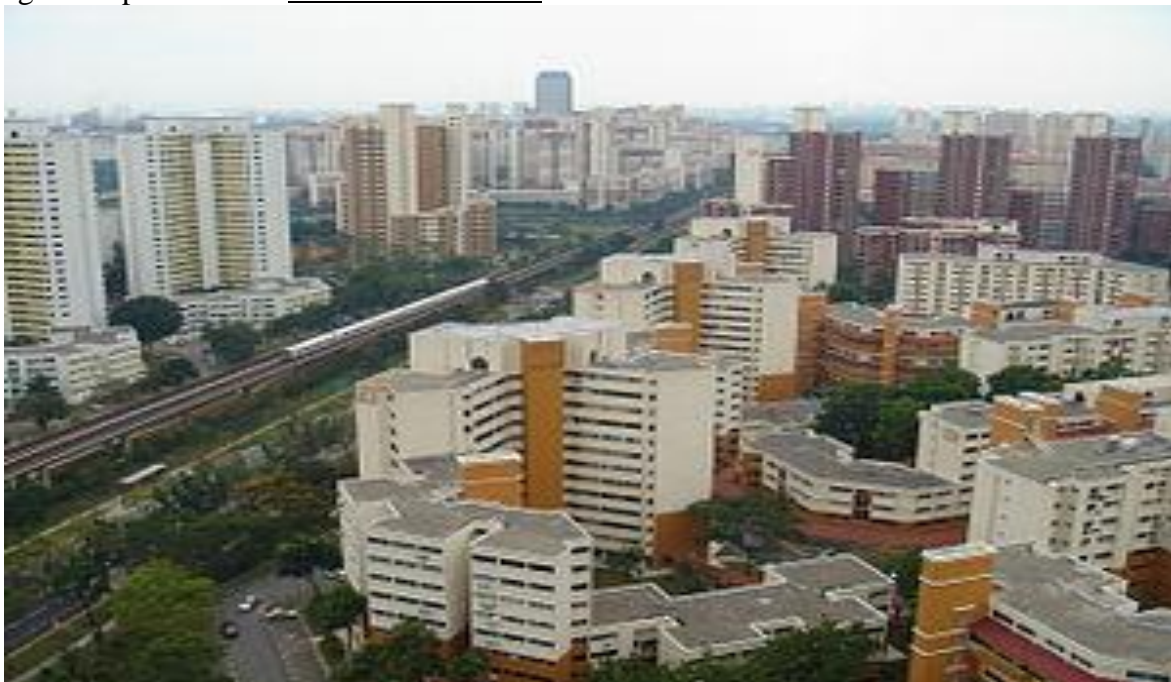
Figure 2: The construction of new towns by the Housing Development Board of Singapore , is an example of planned urbanization
