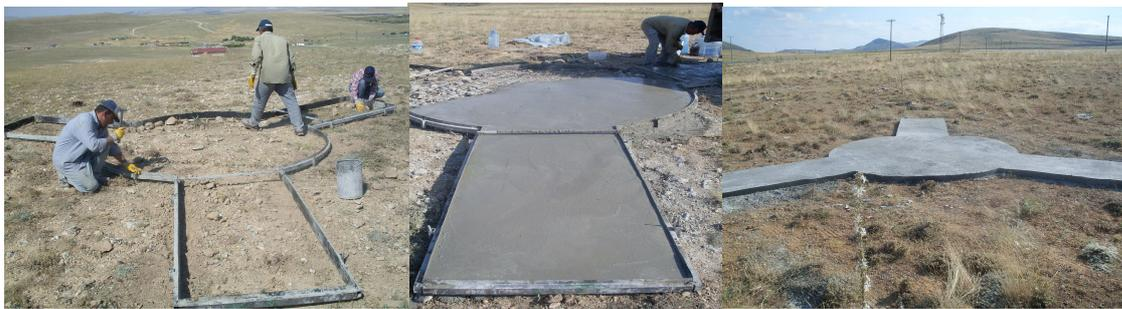
Figure 4.2.2: Poure concrete of GCP on the field.
