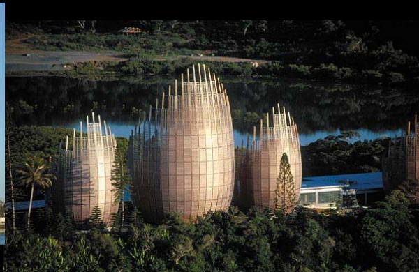
Jean-Marie Tjibaou Cultural Centre, Nouméa, New Caledonia, Renzo Piano architect (1991)
