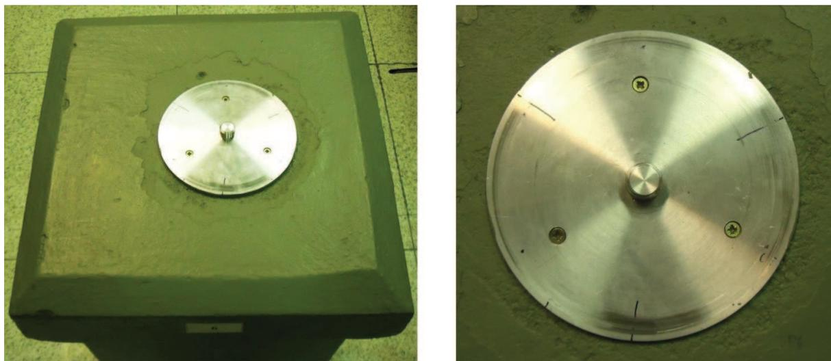
Figure 3 The head of pillar with centring plate
