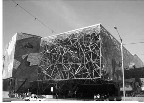
Figure 2. North Atrium showing 14m cantilevered section.
