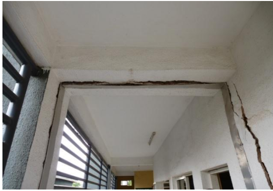
Fig 5: crack around Beams
