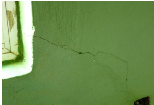
Fig 8: crack in Window
