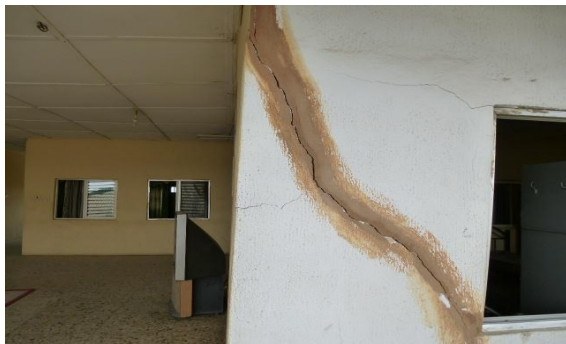
Fig 7: diagonal crack on wall
