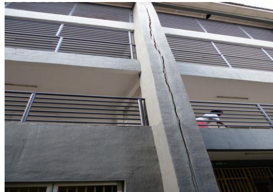
Fig 4: crack along outside Column D4
