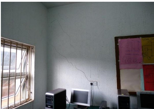
Fig 3: crack in office wall
