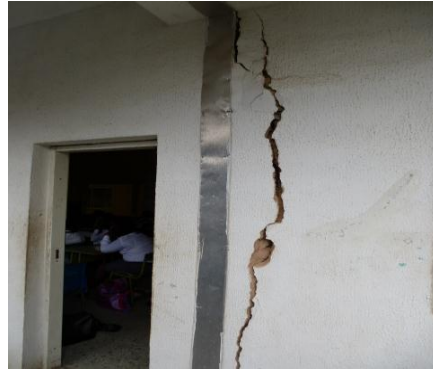
Fig 6: major crack in wall
