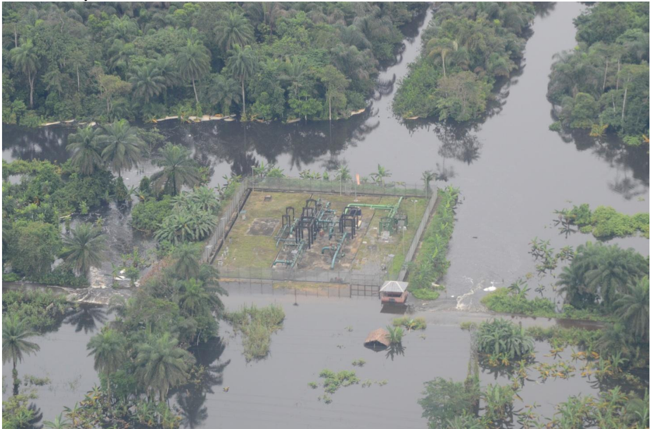
Figure 2: SPDC facility cut-off by flooding, first identified from radar-derived mapping.
