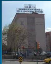
GDLRC Building in Ankara
