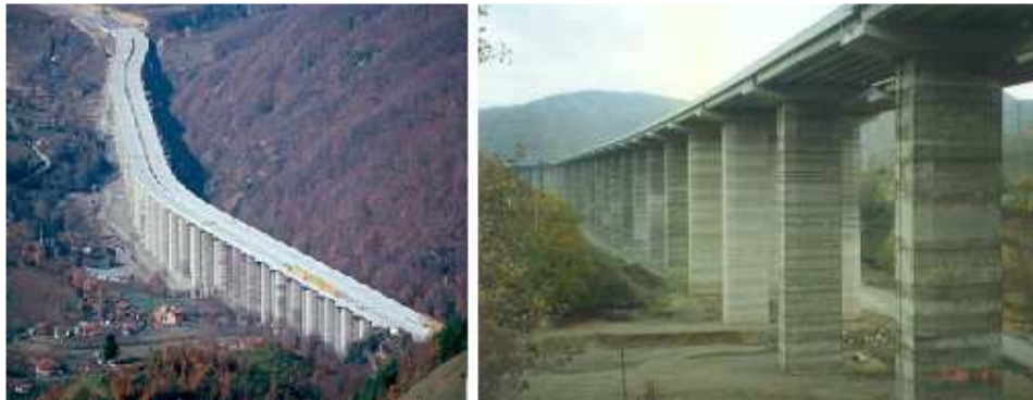
Figure 3 - General view from the Viaduct 1
