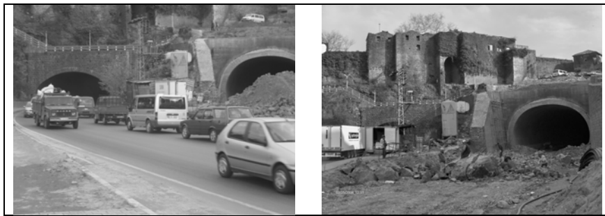
Figure1: Trabzon City Passing Tunnel 2 on KPCR
