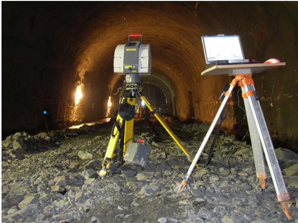
Fig. 1: HDS 3000 laser scanning system
