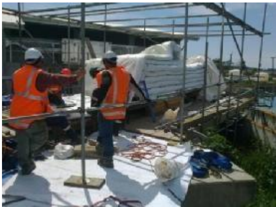
Figure 11: CIPP liner prior to installation
