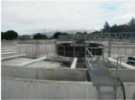
Figure 8: Fully repaired Clarifier 4
