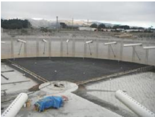
Figure 7: Clarifier 3 floor overlay showing reinforcing mats
