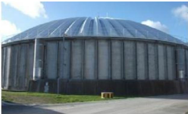
Figure 3: Trickling filter at CWTP
