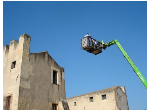
Figure 3: Airborne platform survey
