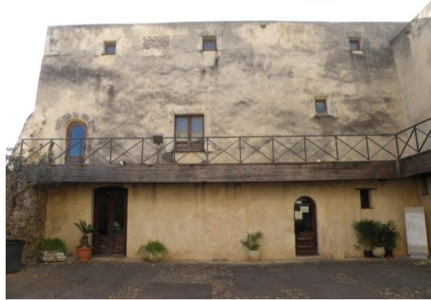
Figure 13: North- East Facade
