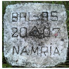
Figure 6: Typical NAMRIA ground control point recovered during the conduct of the GNSS campaign in Bohol.
