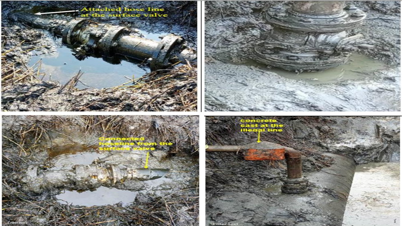
Tapped Point and Illegal Line Connected to the Main Pipeline
