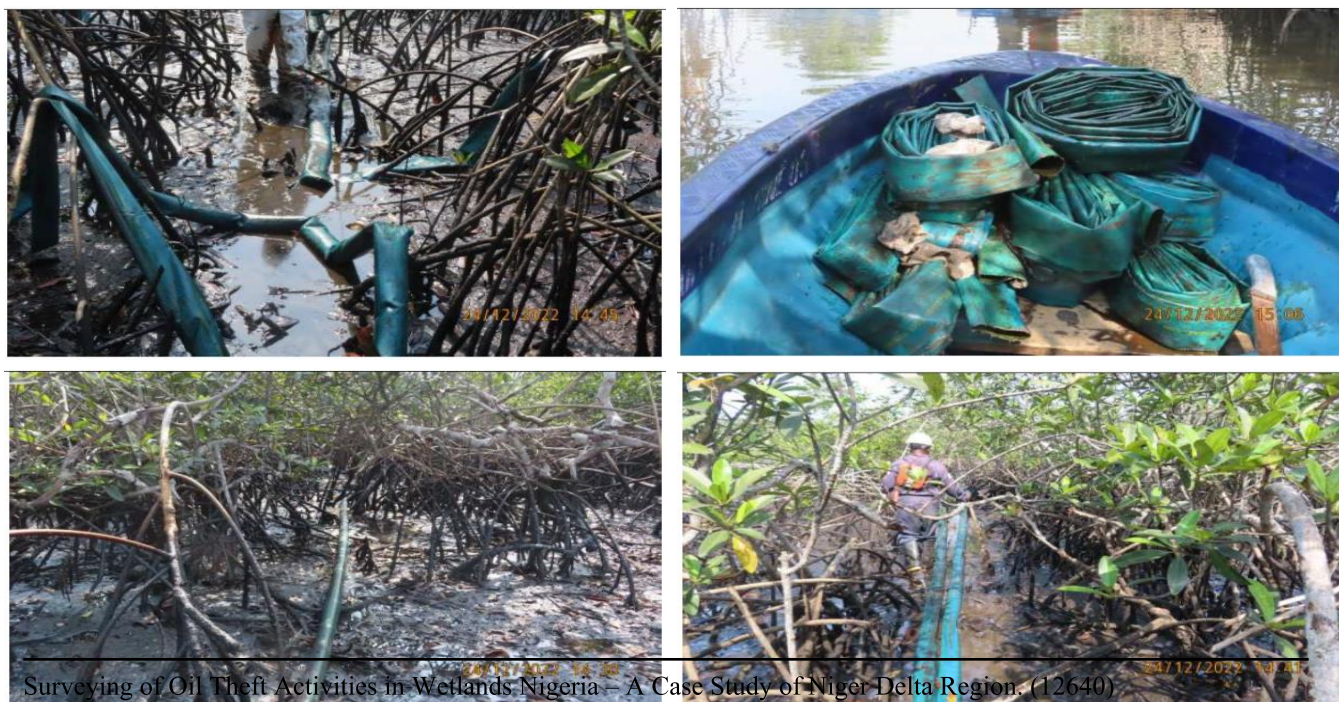
Discovered Siphon Hoses Destroyed During Pipelines ROW Surveillance
