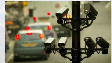
CCTV cameras on roads
