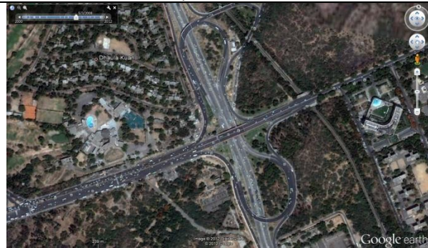
(c) Year 2008- All the road loops completed
