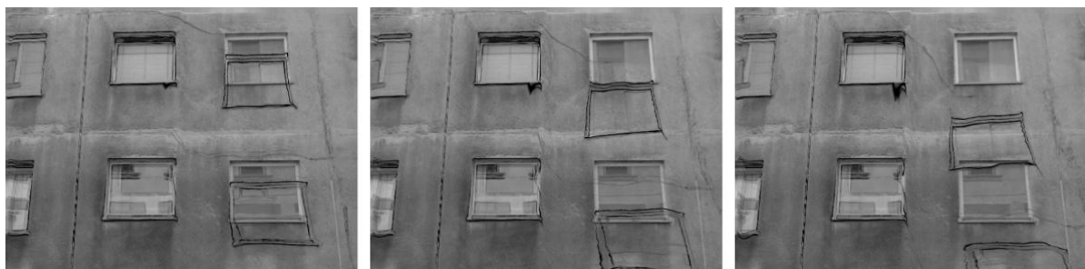
Figure 8: Exaggerated visualization of 2D object deformation. The images of the deformed object are overlaid with the exaggerated versions. The exaggeration parameter is increased from left to right.
